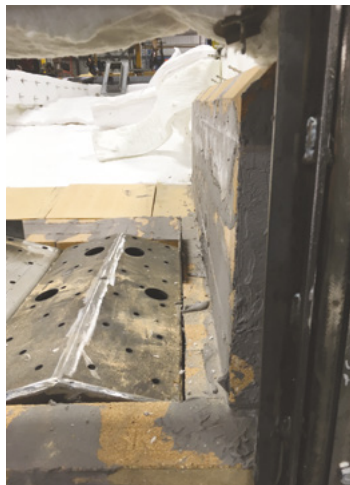
Close-up of the wall
