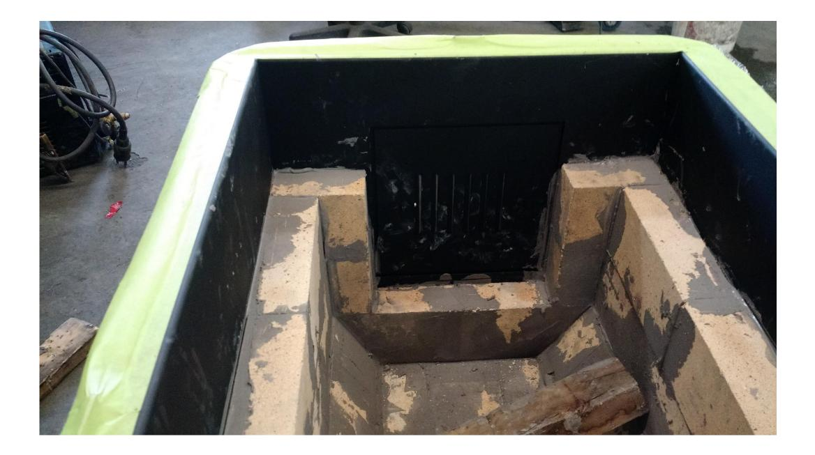
The last row is done with the small bricks 1 ¼ x4 ½ x 9 cut off in such a way as to what does not exceed the height of the evaporator
